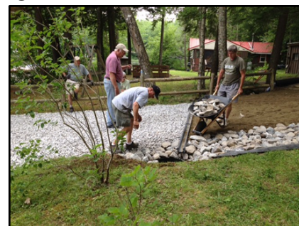
Work at Quimby Lane boat launch
