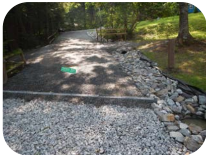
Photo: The newly rebuilt Quimby Lane boat launch was designed to protect the lake from polluted runoff.
