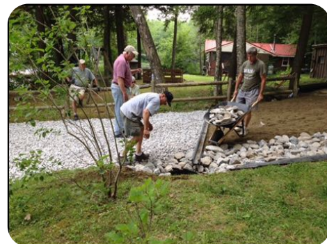
Road association volunteers last July working to rebuild the Quimby Lane boat launch to protect the lake from polluted runoff. This was one of the highest impact erosion sites identified during 30MRWA's watershed survey of Parker Pond in 2011
