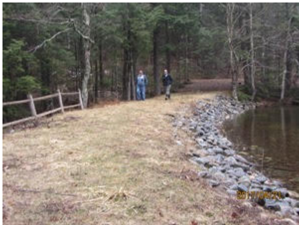
7. Embankment R – Top even - Rip-Rap in place
