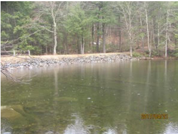
13. Dam right – logs underwater
