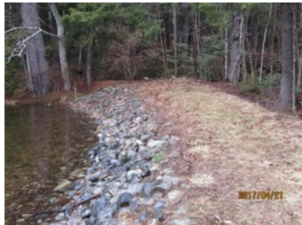
8. Embankment L – Top even - Rip-Rap in place
