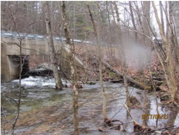
17. BR# 2987 – Small culvert likely
