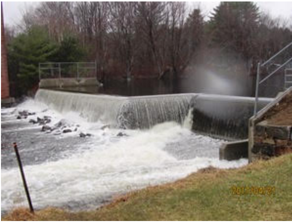
18. Taylor Pond Dam
