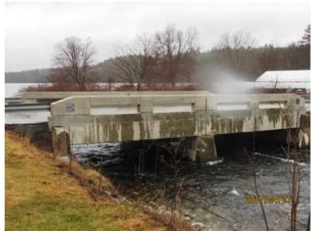
R41 Bridge downstream of Taylor Pond
