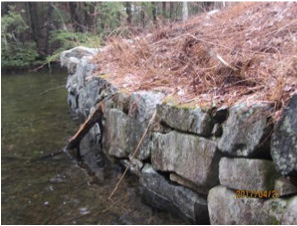
9. Toe L – No erosion or visible movement
