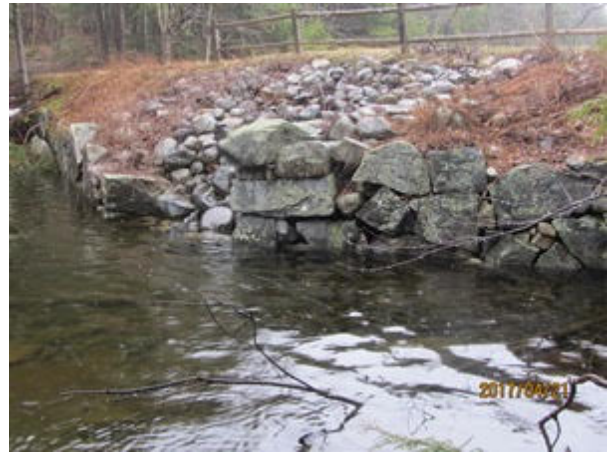
10. Filled-in gateway – insignificant settlement
