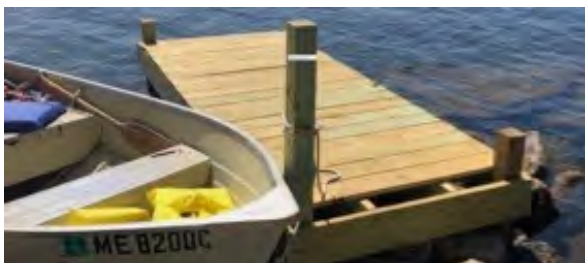
New dock will speed future work
